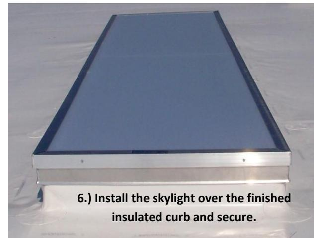
6.) Install the skylight over the finished insulated curb and secure.
