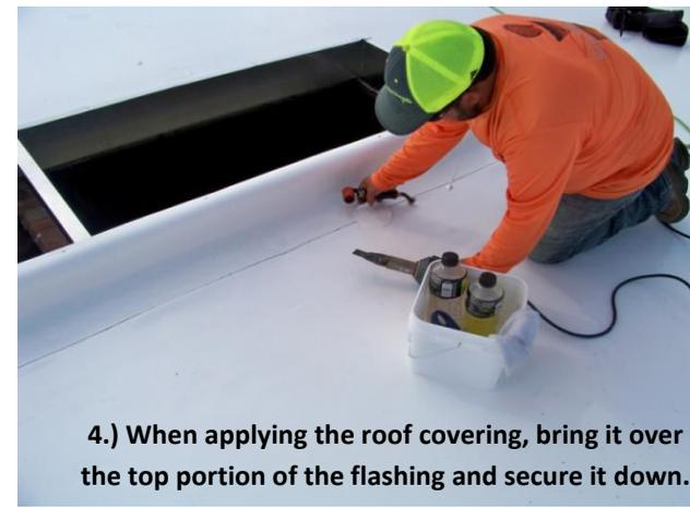
4.) When applying the roof covering, bring it over the top portion of the flashing and secure it down.
