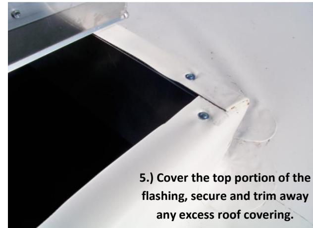
5.) Cover the top portion of the flashing, secure and trim away any excess roof covering.
