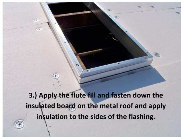
3.) Apply the flute fill and fasten down the insulated board on the metal roof and apply insulation to the sides of the flashing.
