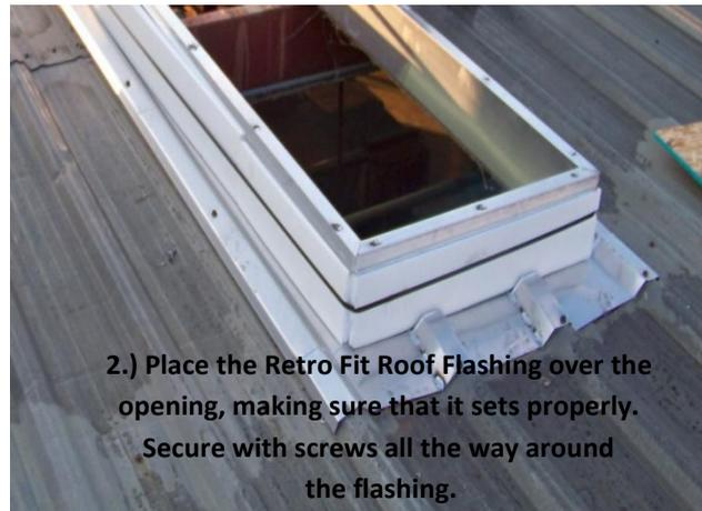
2.) Place the Retro Fit Roof Flashing over the opening, making sure that it sets properly. Secure with screws all the way around the flashing.
