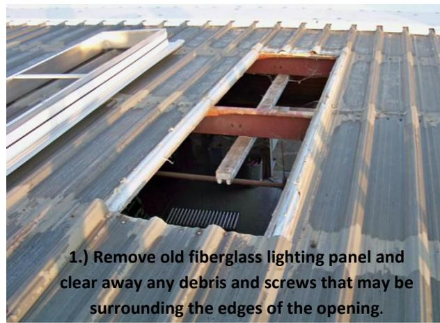
1.) Remove old fiberglass lighting panel and clear away any debris and screws that may be surrounding the edges of the opening.
